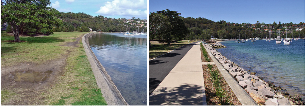
Figure 14 & 15: Pearl Bay, before and after seawall construction
