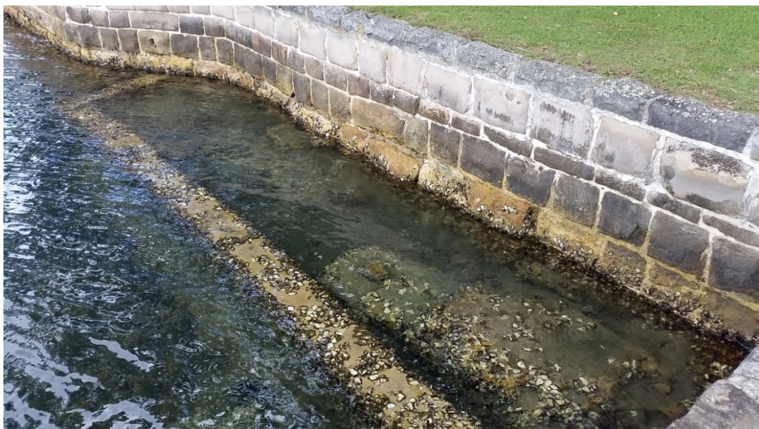
Figure 20: Tidal Pool at Pearl Bay West
