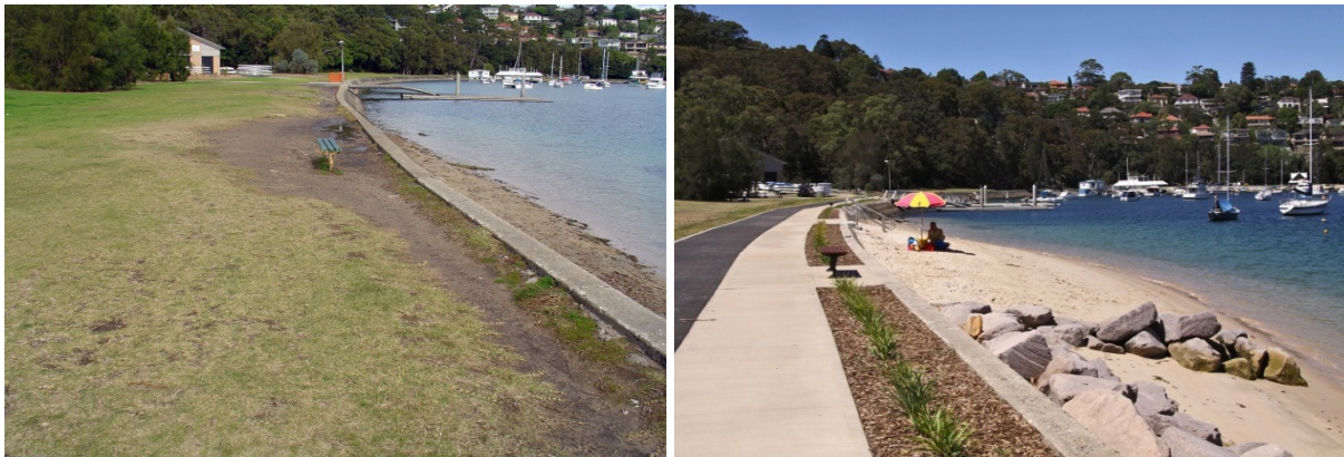
Figure 16 & 17: Pearl Bay, before and after beach reclamation
