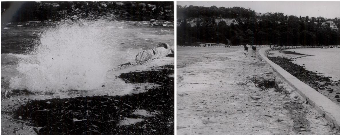
Figure 9 & 10: Historical photos of Pearl Bay, large swells and the 1970's seawall (Mosman Library)
